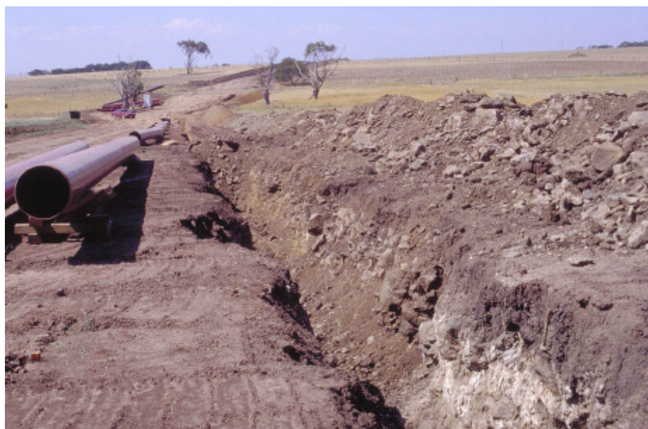
General view towards site SW100, basalt profiles in foreground trench. Note the change in colour of trench spoil across the drainage depression indicating the different provenance of soil parent material.
